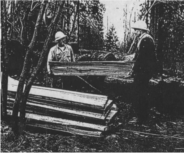
FIGURE 6. Crews worked quickly in the days after the 1962 storm in order to re-open the causeway connector to the Lions Gate Bridge and other park roadways. Images of logging crews in Stanley Park startled observers, who were unaccustomed to witnessing human labour change the landscape of the park. Source: CVA, Photograph Collection, CVA-392-540.
